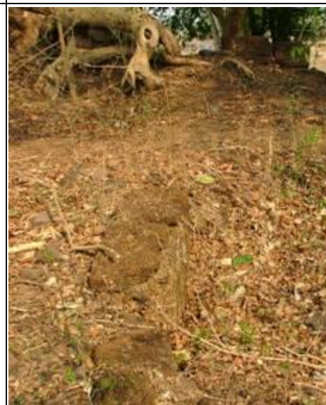
Above: In the eastern part of the structure, there is a depression like a sump inside the temple.
