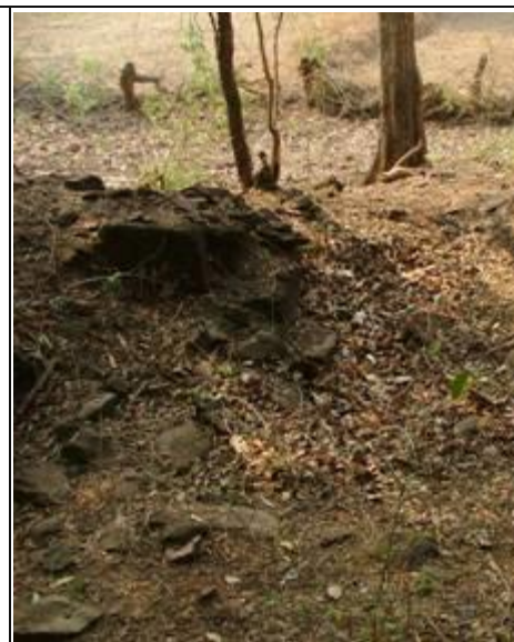
Above: In the southern wall there is an opening assumed to be to the remnants of a door.
