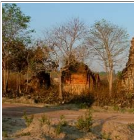
Prasat Bai Baek Buriram Beg. 11th century Left: From west Right: Northern tower from SW
