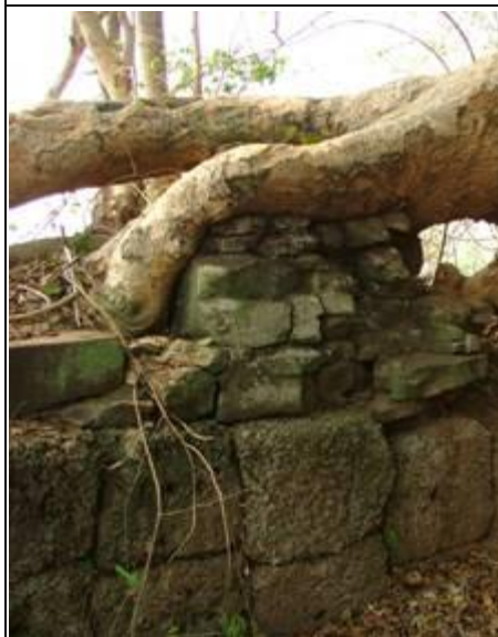
Above: The base of the northern wall indicates that the temple was a sandstone structure on a laterite base.
